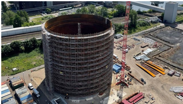
Figure 2. Germany's largest thermal storage tank is 45 m high, 43 m in diameter, and has volume of 56,000 m 3 [5].
