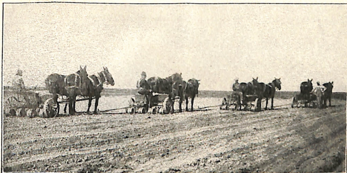
FIG. 1.—PLANTING SUGAR BEET SEED WITH 4-ROW DRILLS, WHEREBY THE SEED SHOULD BE PLACED AT A UNIFORM DEPTH, IN STRAIGHT ROWS, AND IN A FIRM SEED BED.
