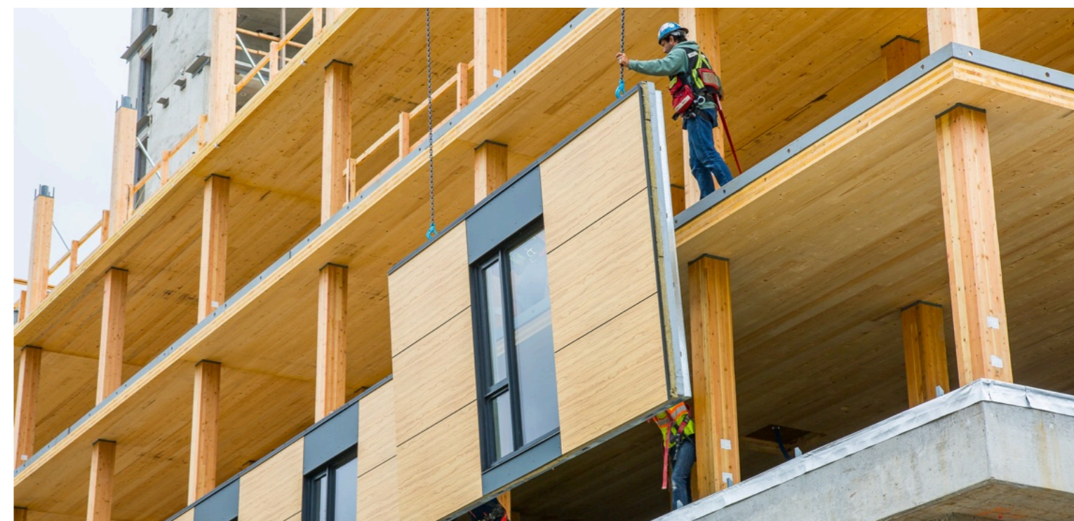
Tallwood House is an 18-storey mass timber hybrid student residence at the UBC Vancouver campus. © Living Labs UBC, https://livinglabs.ubc.ca/projects/brock-commons-tallwood-house
