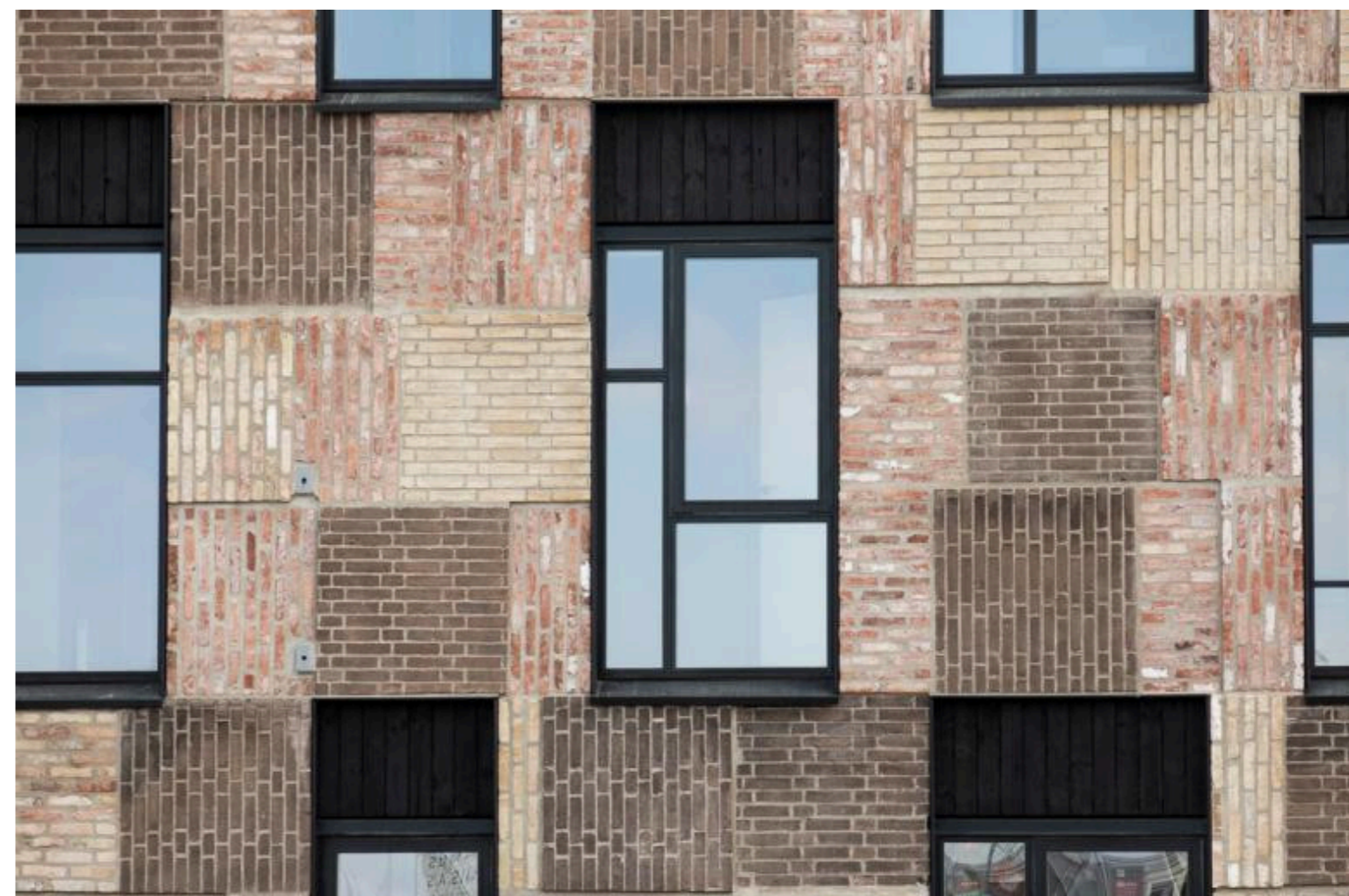
The brick modules at the Resource Rows in Copenhagen were cut out of old buildings at the Carlsberg Brewery. Lendager Group, 2019, Photo © Lendager
