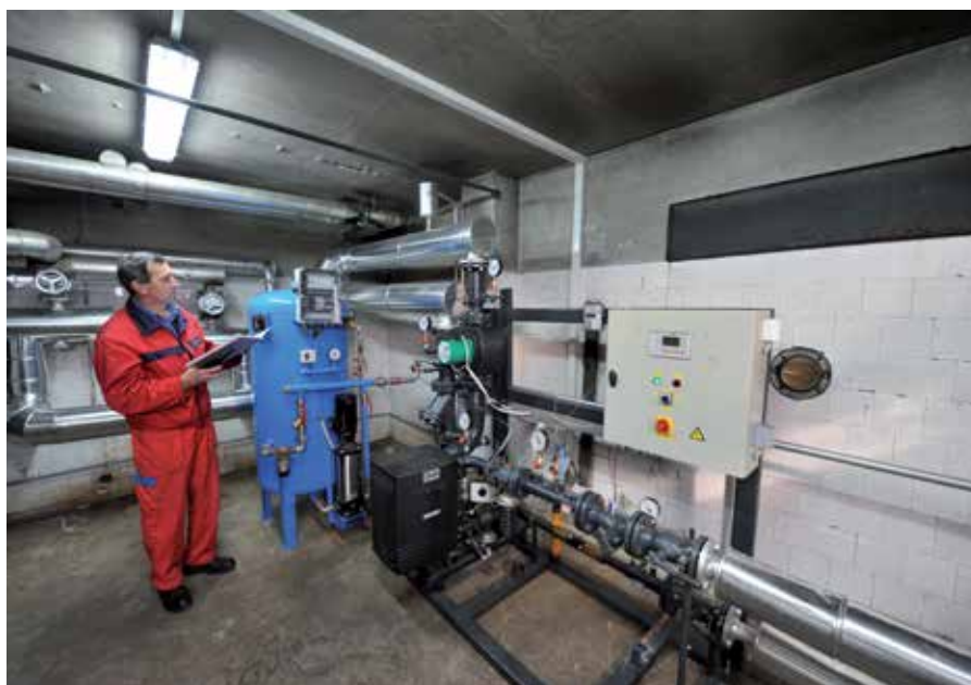
The boiler room under a 15-story building in central Tuzla: An employee from Centralno Grijanje checks and notes down data of consumption and variations in temperature between this new Danfoss substation and the building. It is a huge improvement of life quality for the residents.
